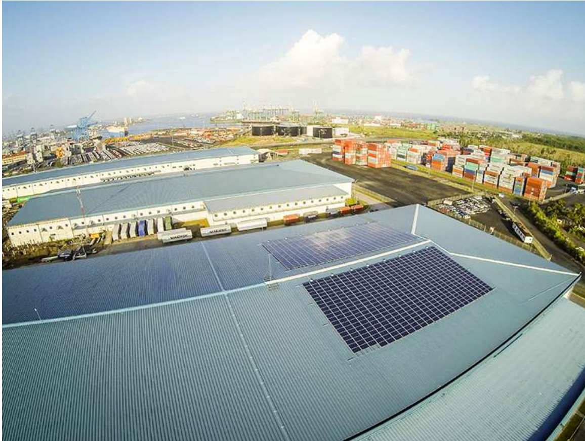
Source: PLAT Installs Solar Panels at Warehouse in Colon Free Zone in Panama, https://www.panasonic.com/caribbean/corporate/news
